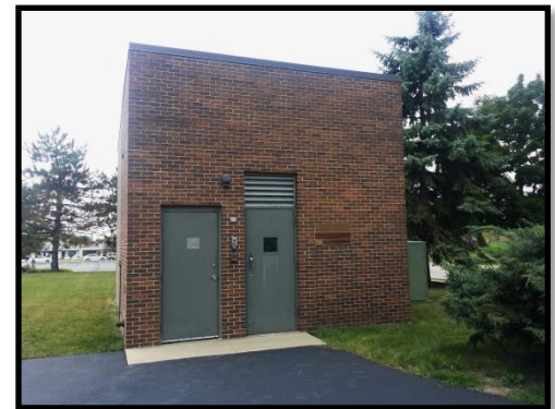
Figure 9-2 Well House #1 Exterior
