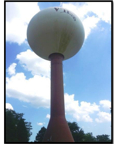
Figure 9-1 Hawthorn Water Tower
