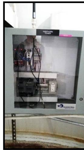
Figure 9-6 Existing Well House Control Panel
