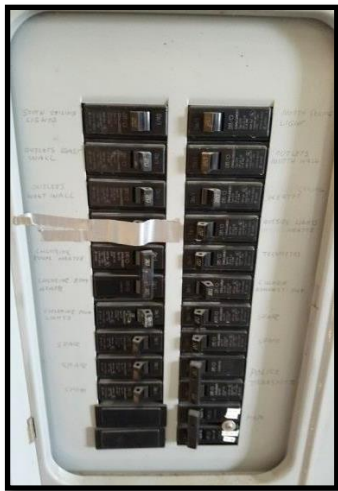
Figure 9-4 Well House #1 Existing Lighting Panel
