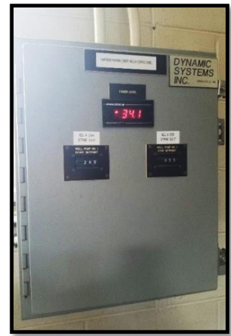
Figure 9-7 Existing Well House Telemetry Panel
