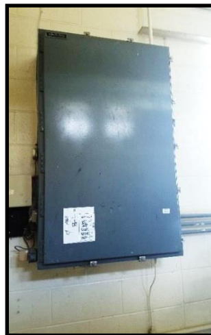
Figure 9-5 Existing Tower SCADA Panel
