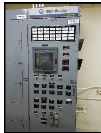
Figure 5-4 Existing Greggs Landing Reservoir Control Panel
