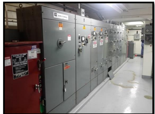
Figure 4-3 Existing MCC in the Hawthorn Center Reservoir Pumping Station
