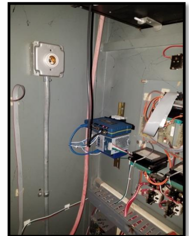
Figure 4-7 Existing Hawthorn Center Reservoir Control Panel Interior
