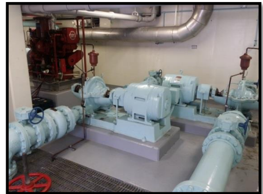
Figure 4-2 Existing 1,500 gpm Water Supply Booster Pumps
