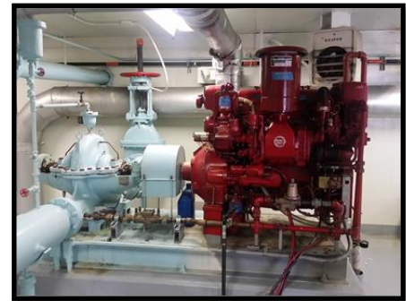
Figure 4-4 Existing 1,500 gpm Diesel-Driven Fire Pump
