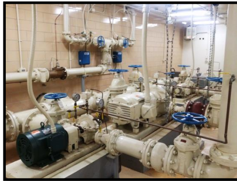
Figure 10-2 Water Supply Booster Pumps
