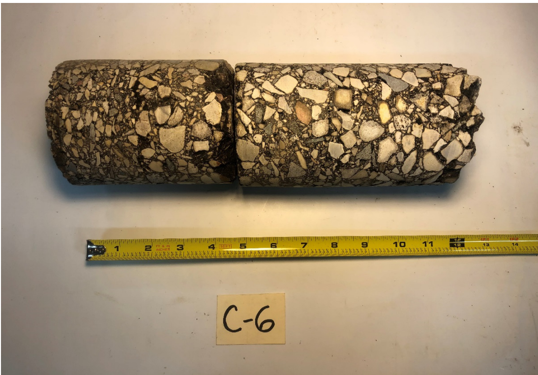
Pavement Core C-6: Catalpa Drive
