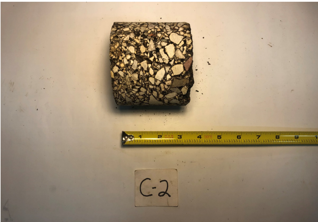
Pavement Core C-2: W. Columbia Bay Road
