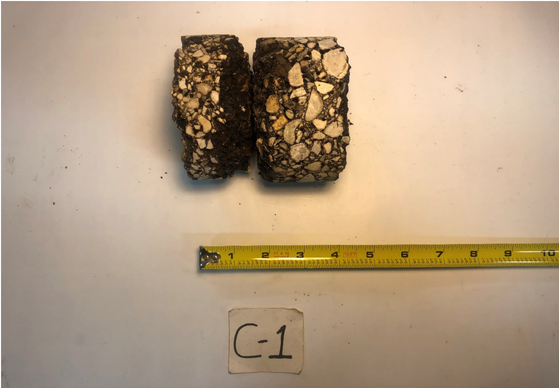
Pavement Core C-1: W. Columbia Bay Road
