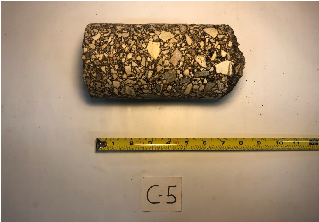
Pavement Core C-5: Hilltop Road
