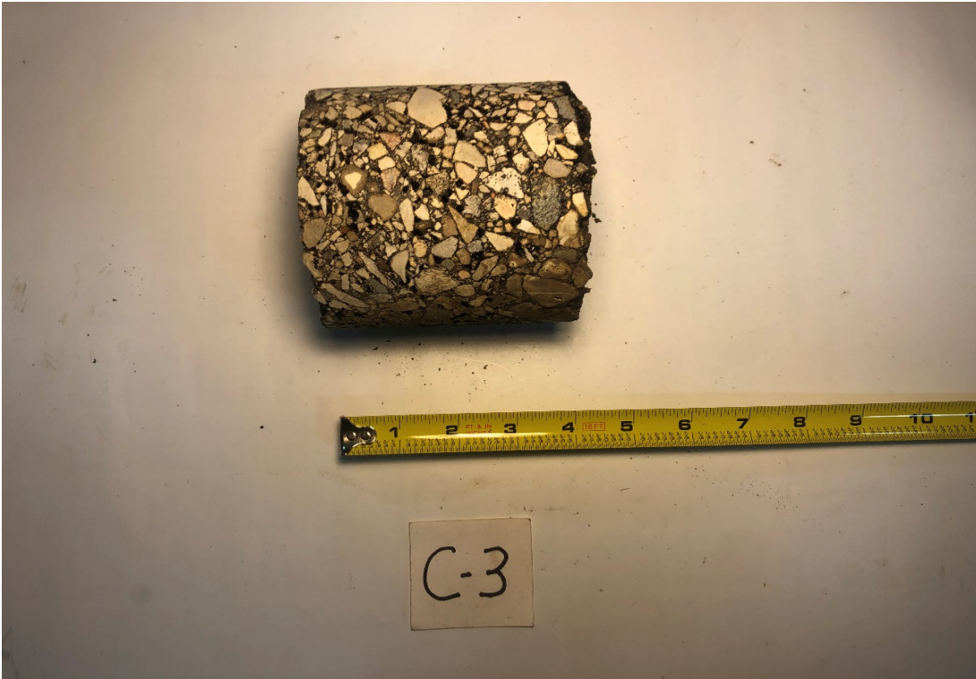
Pavement Core C-3: W. Columbia Bay Road
